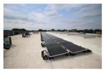
The project consisted of 70KW of ballasted, roof mounted solar panels tied to two (2) Sol-Ark 30K inverters. The battery system is 40kWh of Deka batteries, which back up a subpanel of the owner's critical loads. An interior LED lighting retrofit was also completed to lower power usage on the critical circuits and extend backup battery duration.
