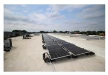
The project consisted of 70KW of ballasted, roof mounted solar panels tied to two (2) Sol-Ark 30K inverters. The battery system is 40kWh of Deka batteries, which back up a subpanel of the owner's critical loads. An interior LED lighting retrofit was also completed to lower power usage on the critical circuits and extend backup battery duration.
