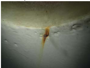
Interior Manway #2 Photo of corrosion
