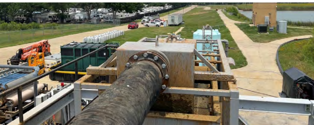
Elm Fork - Dewatering Site and Office
