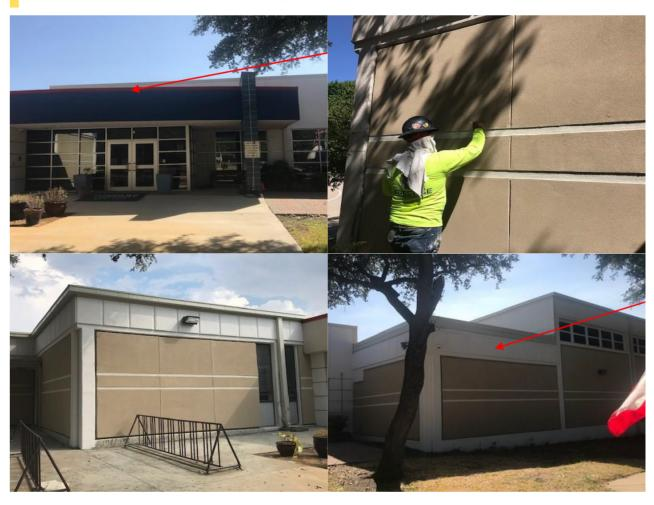
Shepard Elementary School Façade Renovation: New EIFS system, exterior walls coating, exterior vertical joints, waterproofing and glazing, new metal copings.
