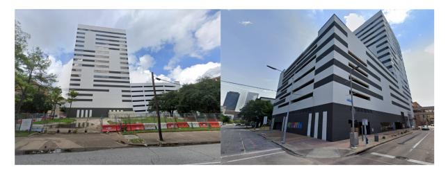
ST. Joseph Medical Center: Exterior Facade Renovation: Remove and Install new expansion joints, engineering, pedestrian safety, exterior coating wall and metal surfaces
