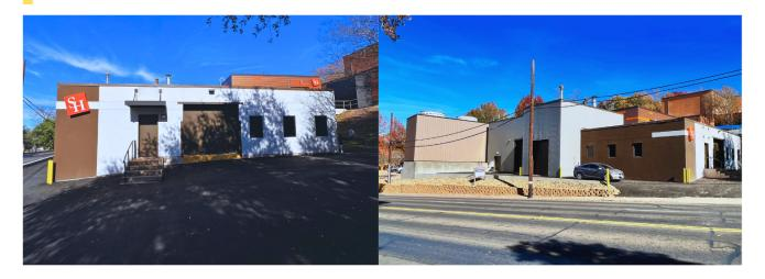
SHSU West Plant Façade Renovation: Existing EIFS system demolition, faux windows installation, existing awning demolition, new EIFS system, new awning installation, metal panel buildings coating
