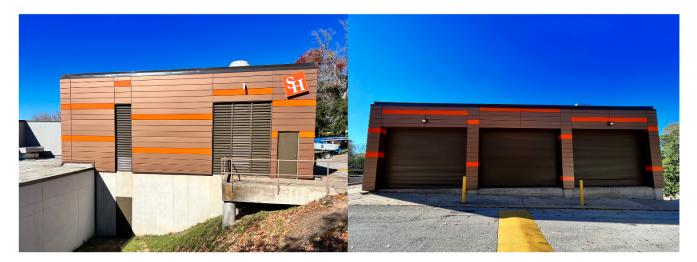
SHSU West Plant Façade Renovation: Metal panels demolition, insulation, new metal framing, sheathing, waterproofing, new metal copings, new metal panels system
