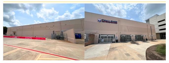
Houston Community College West Loop Campus: Prep and Paint Building Envelope (walls, downspouts, door and window frames) Metal Awning, Metals, Light Poles and Bases, Roof Gas Pipes
