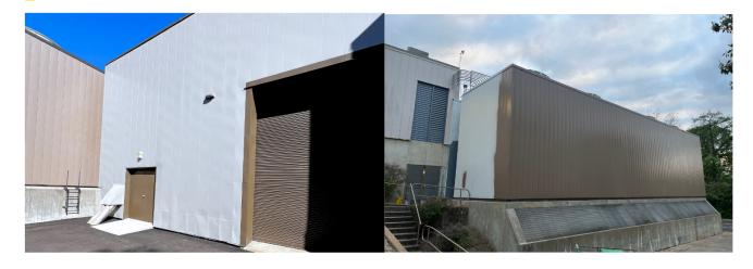
SHSU West Plant Façade Renovation: Pressure wash, prep, prime and coating
